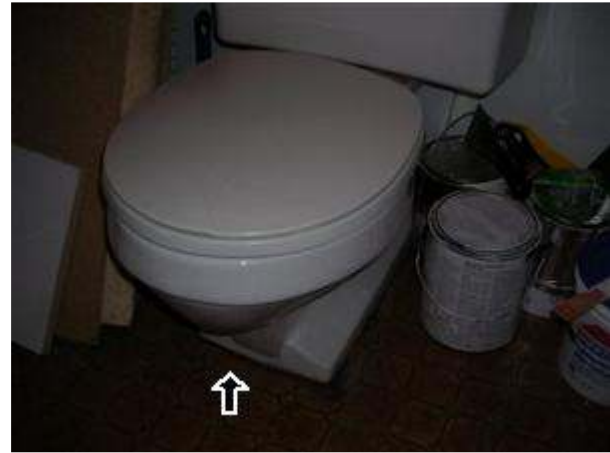
5.6.D Picture 1 Shower valve leaking/ damage around tub/shower unit 5.6.D Picture 2 Toilet leaking at the base unit
