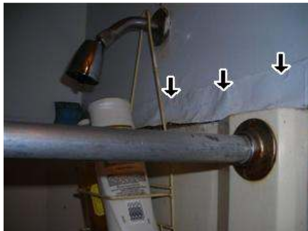
5.6.C Picture 2 Evidence of prior leaks.
