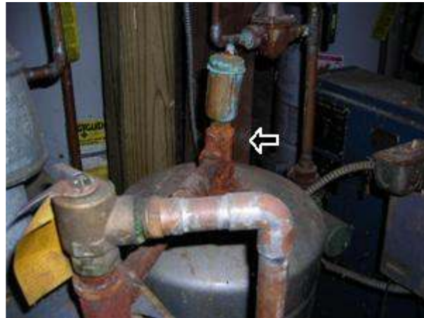
5.17.D Picture 1 Pressure relief valve not installed correctly 5.17.D Picture 2 Corrosion at expansion tank
