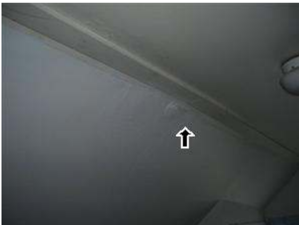
5.0.D Picture 1 Ceiling repair. Typical throughout the building
