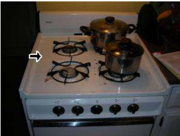
5.11.A Picture 1 Burners do not lite automaticaly
