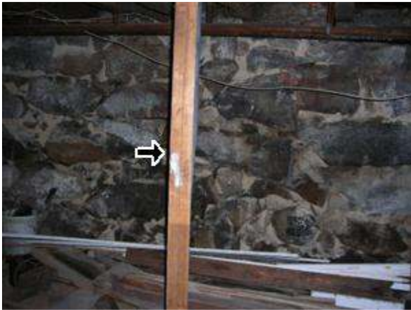
3.2 Picture 1 Wood collum should be larger or replaced with steel lally collums
