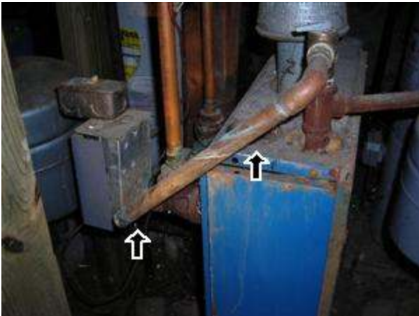
5.17.D Picture 1 Pressure relief valve not installed correctly 5.17.D Picture 2 Corrosion at expansion tank
