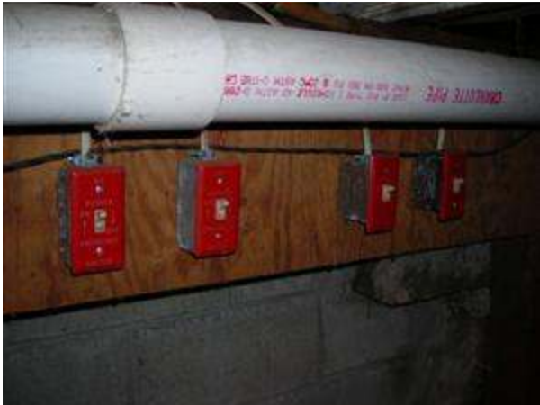
3.0 Picture 3 Emergency shut off switches for the heating systems are in the basement.
