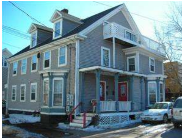
Front view of building
