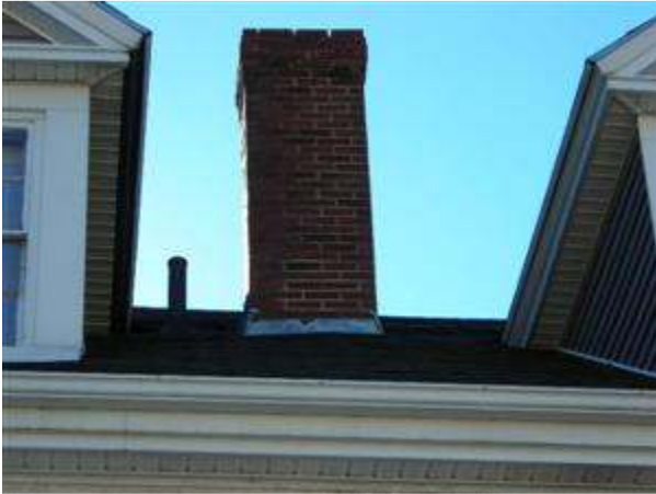
1.2 Picture 1 Some repointing may be required, front chimney
