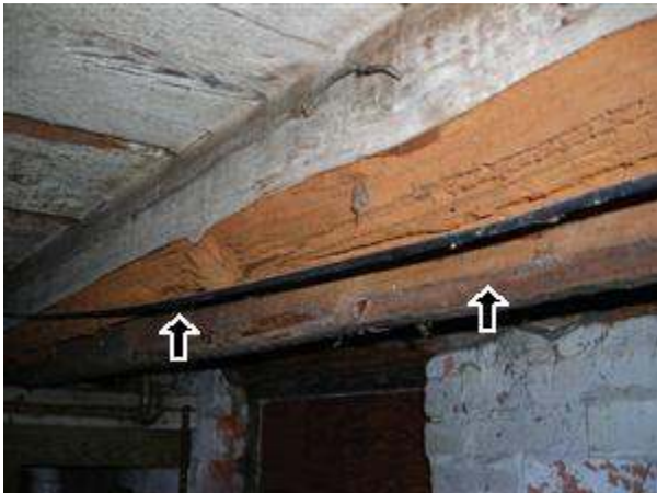
3.3 Picture 1 Past insect damage/repairs
