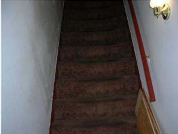
5.16.D Picture 1 Stair leading to 19B
